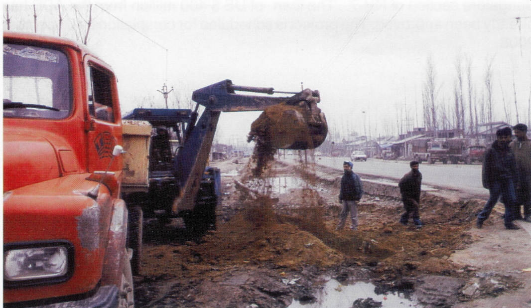
Work in progress on Srinagar Bypass
