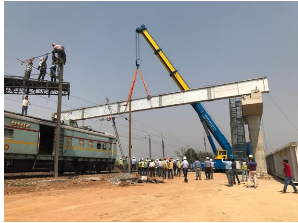
(d) Photo: Crossing of girder across track
