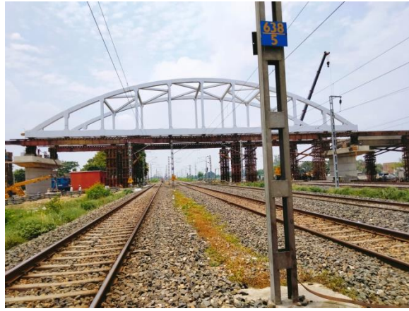
(g) Photo: Bringing BSG to its final location over piers
