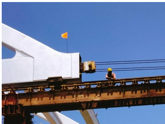
(e) Photo: Fixing Winch and rope assemblies
