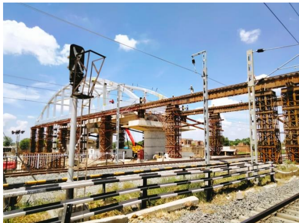
(d) Photo: Completing Temporary arrangements for launching
