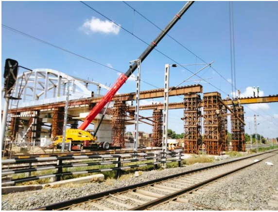
(a) Photo: Erection of temporary arrangements- Trestles
