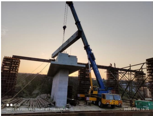
(a) Photo: Erecting temporary arrangements
