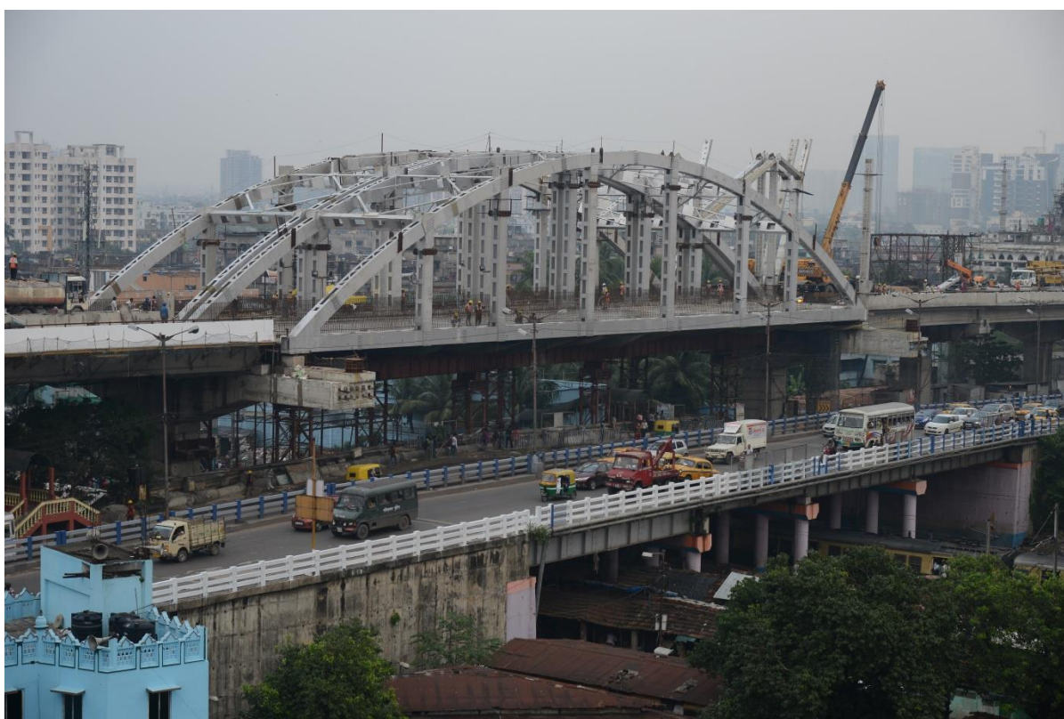
Fig 1 Photo: View of Bow String Arch Girder during construction stage (Park Circus station of Eastern Railway)
