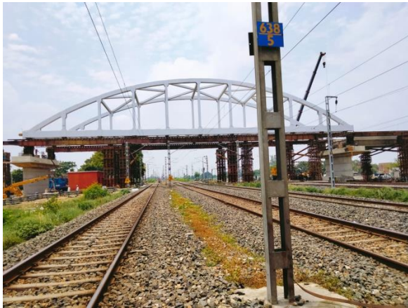
(a) BSG positioned over piers with temporary arrangements in place
