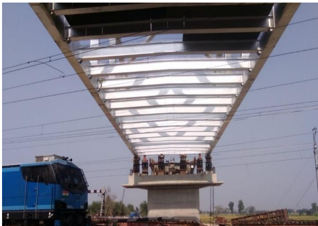
(a) Photo: Arrangement of temporary support for lowering
