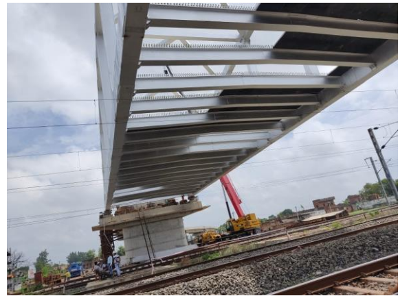
(d) Clearing of site after removal of all ground arrangement
