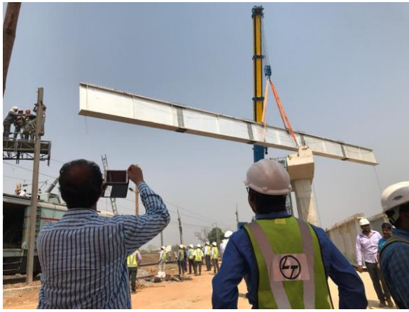
(c) Photo: Lifting of girder
