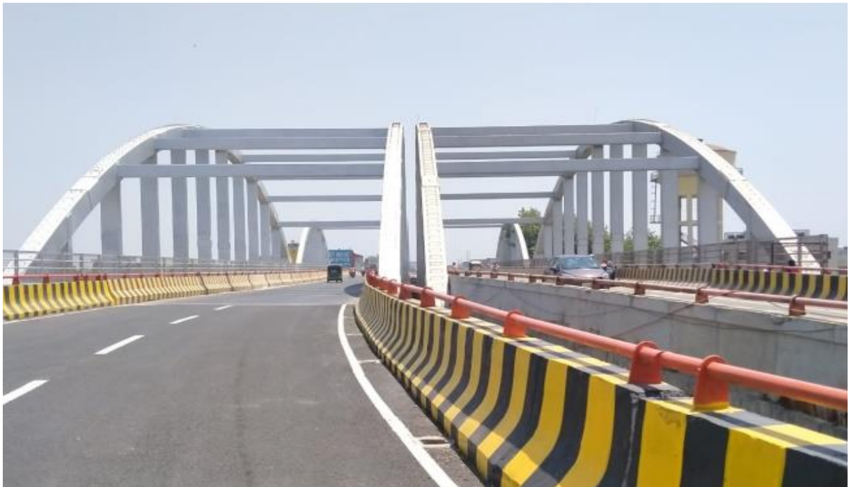
Fig. c): Bow String Arch Steel Girder
