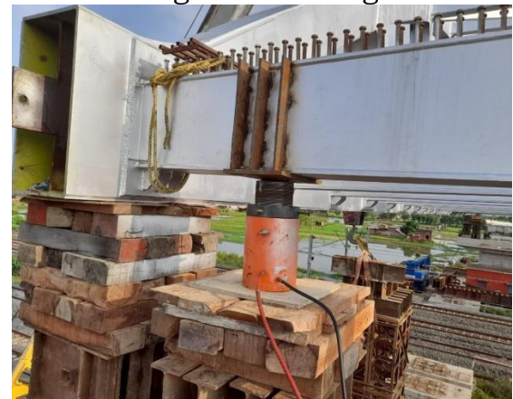
(b) Photo: Jacking arrangement below End Cross Girder
