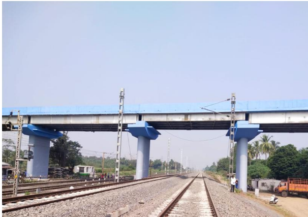
Fig. a): Composite Steel Plate Girder
