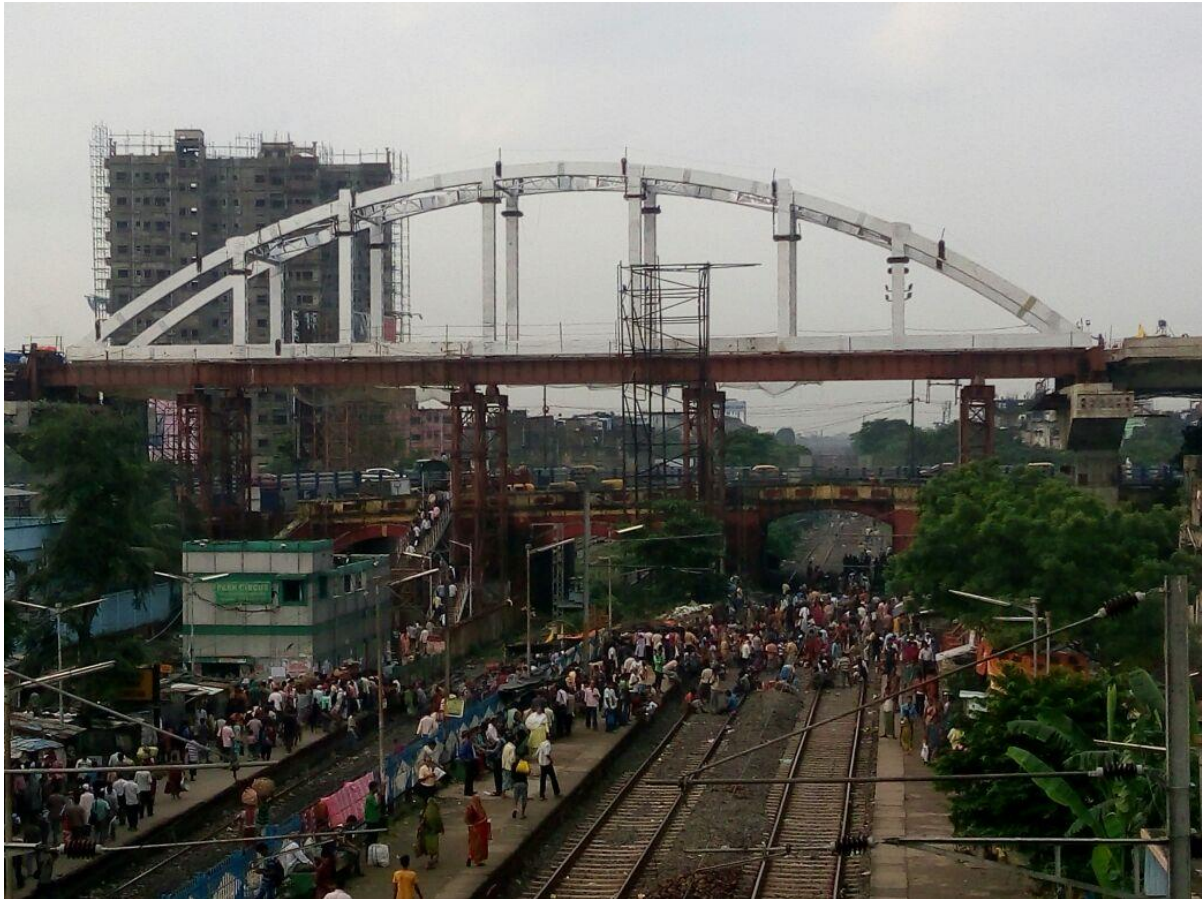
Fig 2 Photo: View of Bow String Arch Girder from Railway Station during construction stage (Park Circus station of Eastern Railway)
