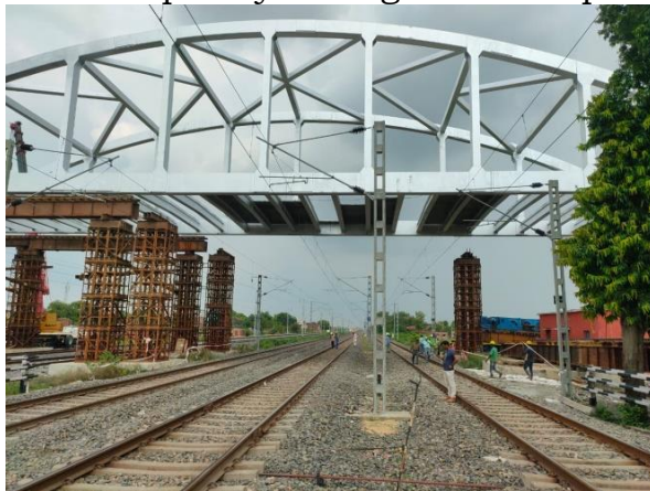
(c) Supporting of BSG over piers and removal of beams continued
