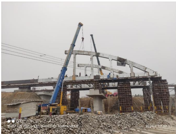
(c) Photo: Completing the sequence from one end to the other
