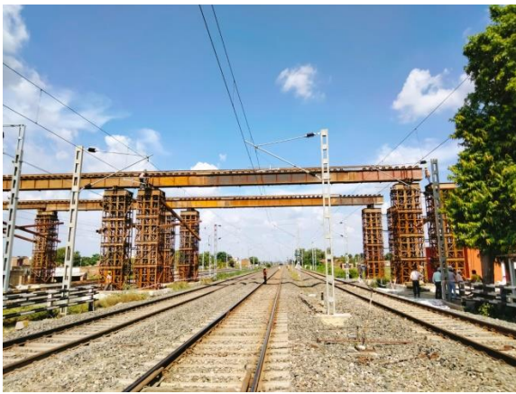
(c) Fixing longitudinal beams and Trestles
