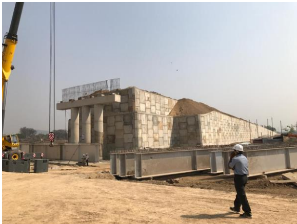
(a) Photo: Assembled girders to be brought near the crane
