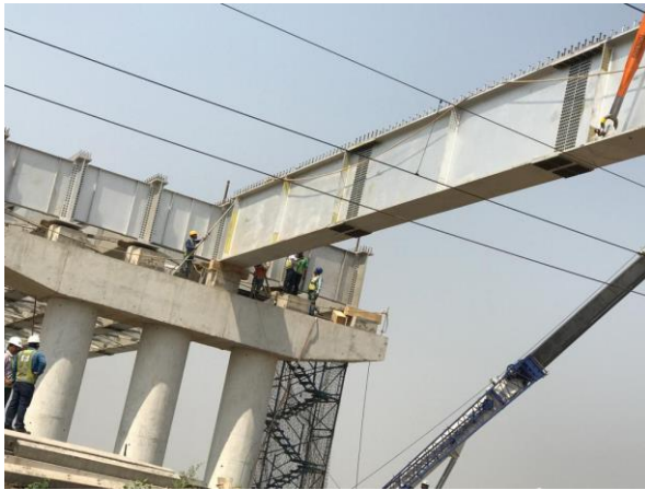
(e) Photo: Placing of girder in position
