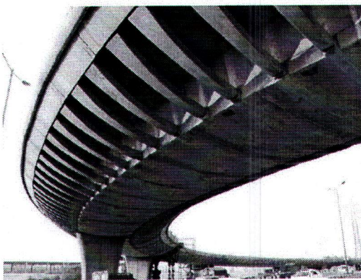
Fig. a Cantilevers of wide deck supported by struts
