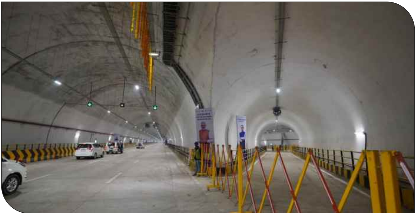
Rewa-Sidhi Tunnel on NH 24, inaugurated by Hon'ble Minister (RT&H)
