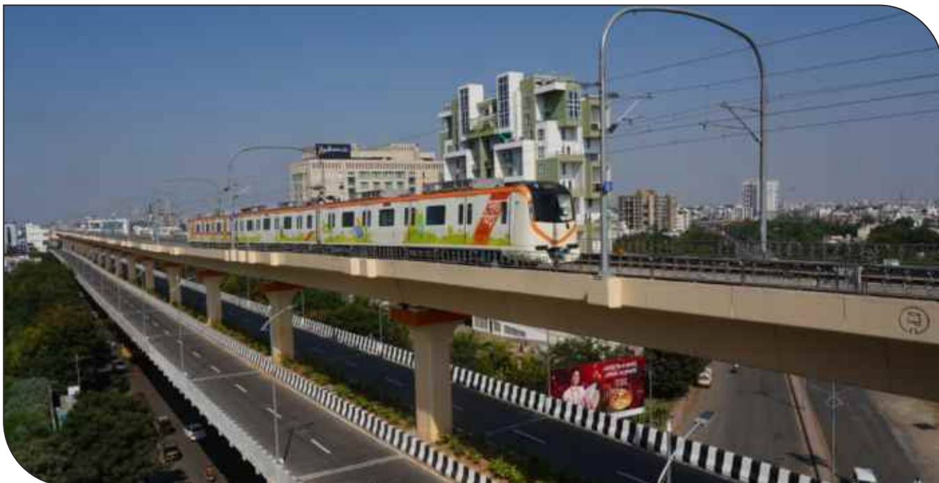
Longest Double Decker Viaduct with Highway Flyover & Metro Rail in Nagpur.
