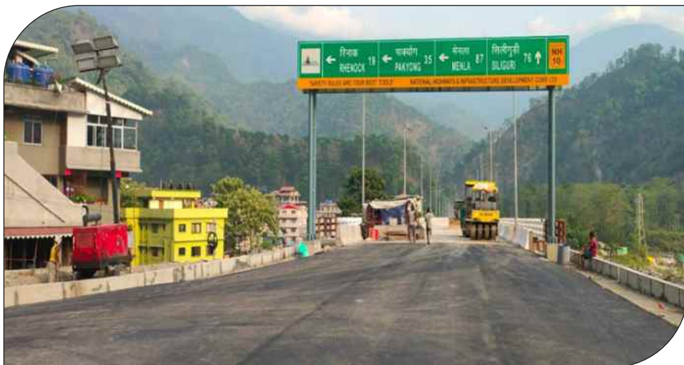
Construction of Rangpo Viaduct Connecting Sikkim with West Bengal
