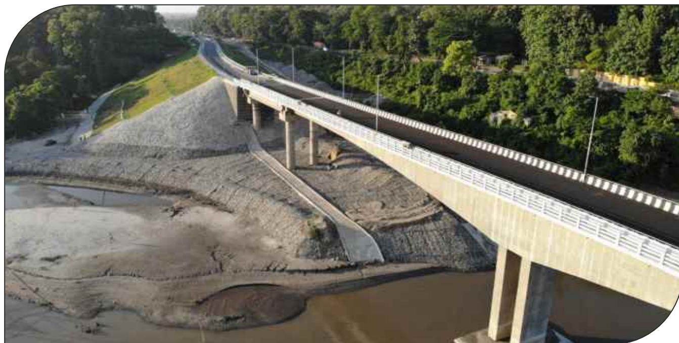
Kaliabor - Tainali Bridge Assam
