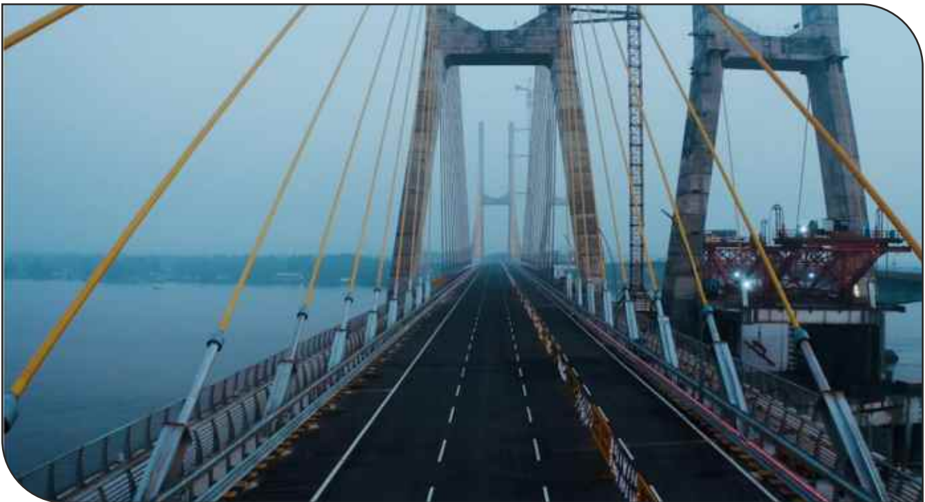
Zuari Bridge, Goa
