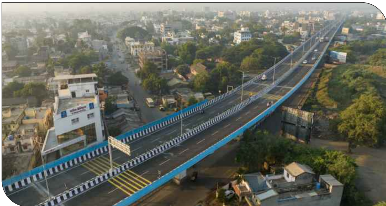
Elevated Structure (Flyover) in Ahmednagar City
