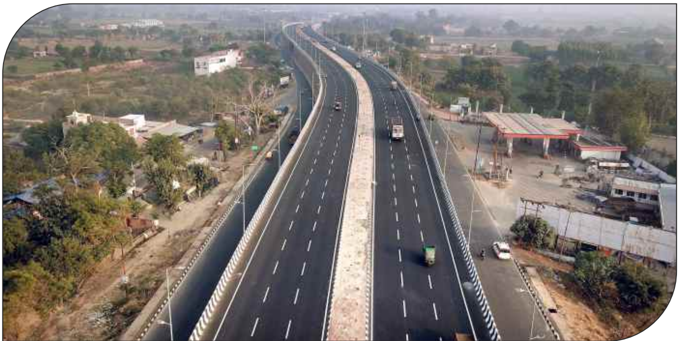
Agra - Etawah Bypass Section of NH-3
