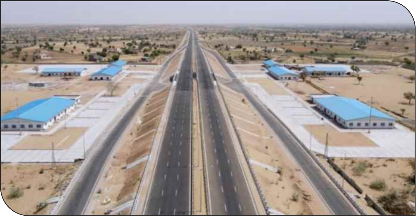
Rasisar Deoghar Greenfield Highway Project (Rajasthan)
