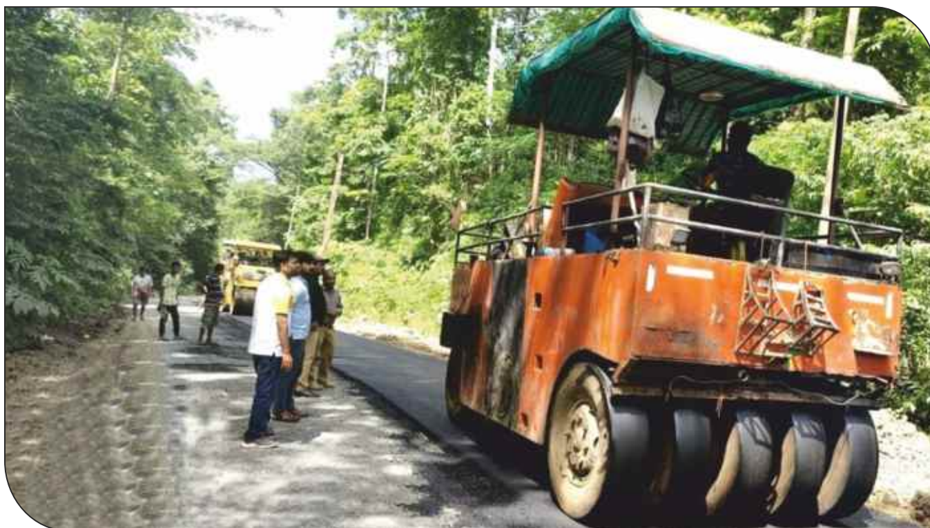
Checking of BC Laying And Rolling at Andman & Nicobar Islands
