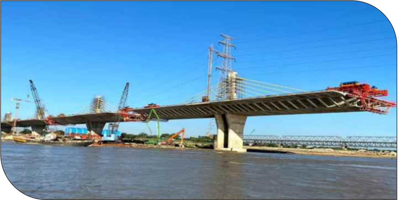
Construction of Aunta Simariya Project including Ganga Bridge with approach Roads on NH 31
