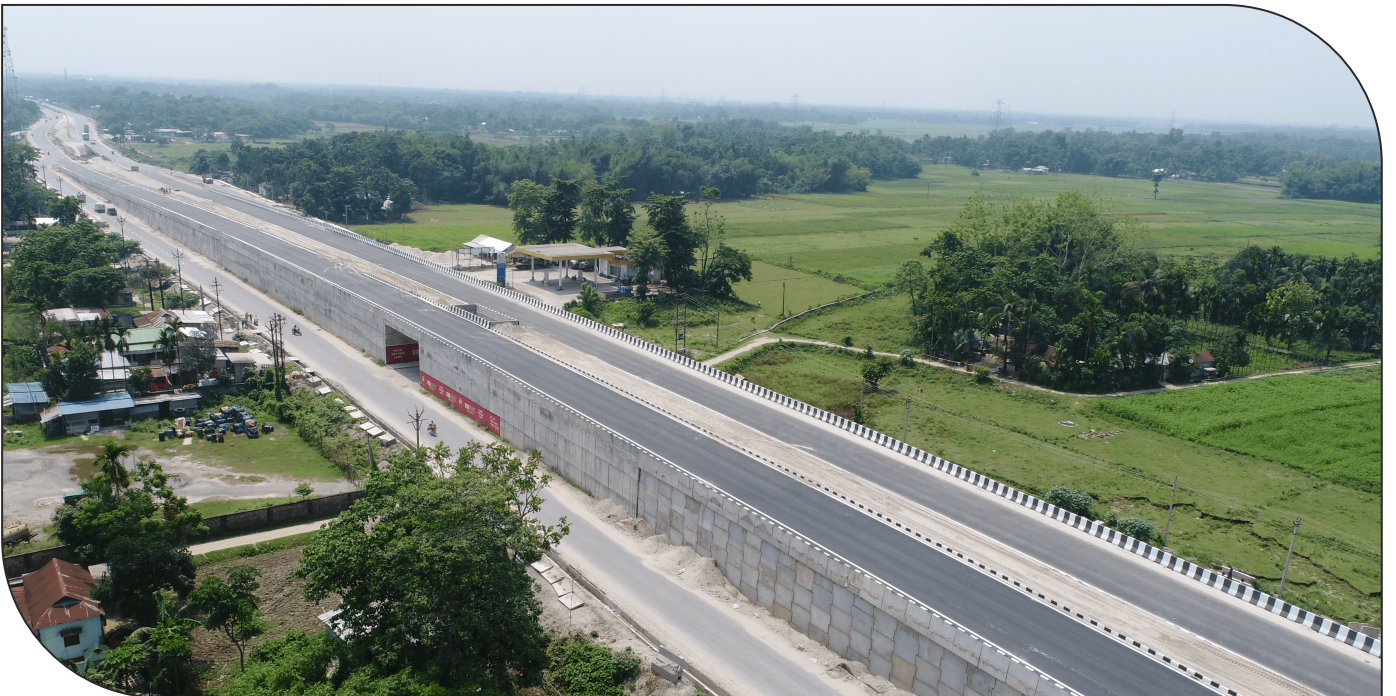
Ghoshpukur - Dhupguri Section of NH 31D
