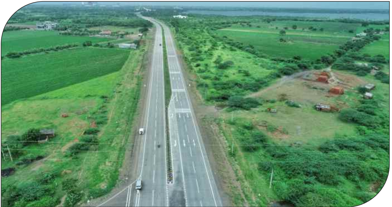
Dwarka-Khambhaliya-Devariya Section of NH-151A
