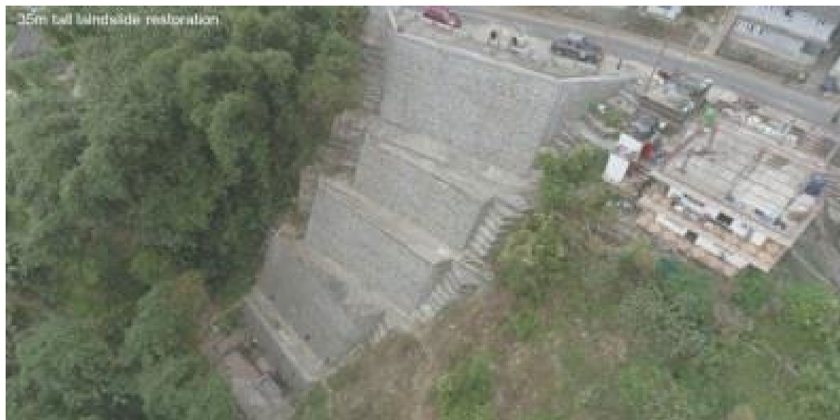
Completed Restoration Work for Valley Slope at "Tindharia I" on NH55
