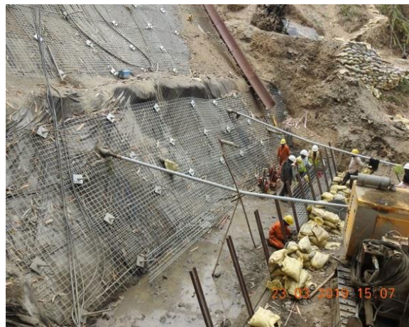
Base level of TerraLink® structure before start of filling and compaction
