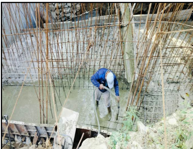
CONCRETING WORK FOR RCC R/WALL AT HOME BANK OF CHUNGTHANG BRIDGE ON G-C
