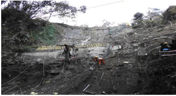
Activity of surface cleaning, drilling, fixing of welded wire back mesh simultaneously with soil nailing of existing valley slope at “Tindharia I”
