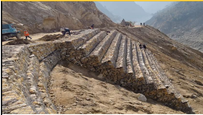
CONSTRUCTION OF R/S/WALL AT KM 7.552 TO KM 7.560 on Ln-K road
