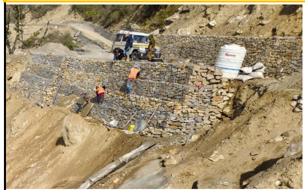
CONSTRUCTION OF R/S/WALL AT KM 7.544 TO KM 7.552 on Ln-K road
