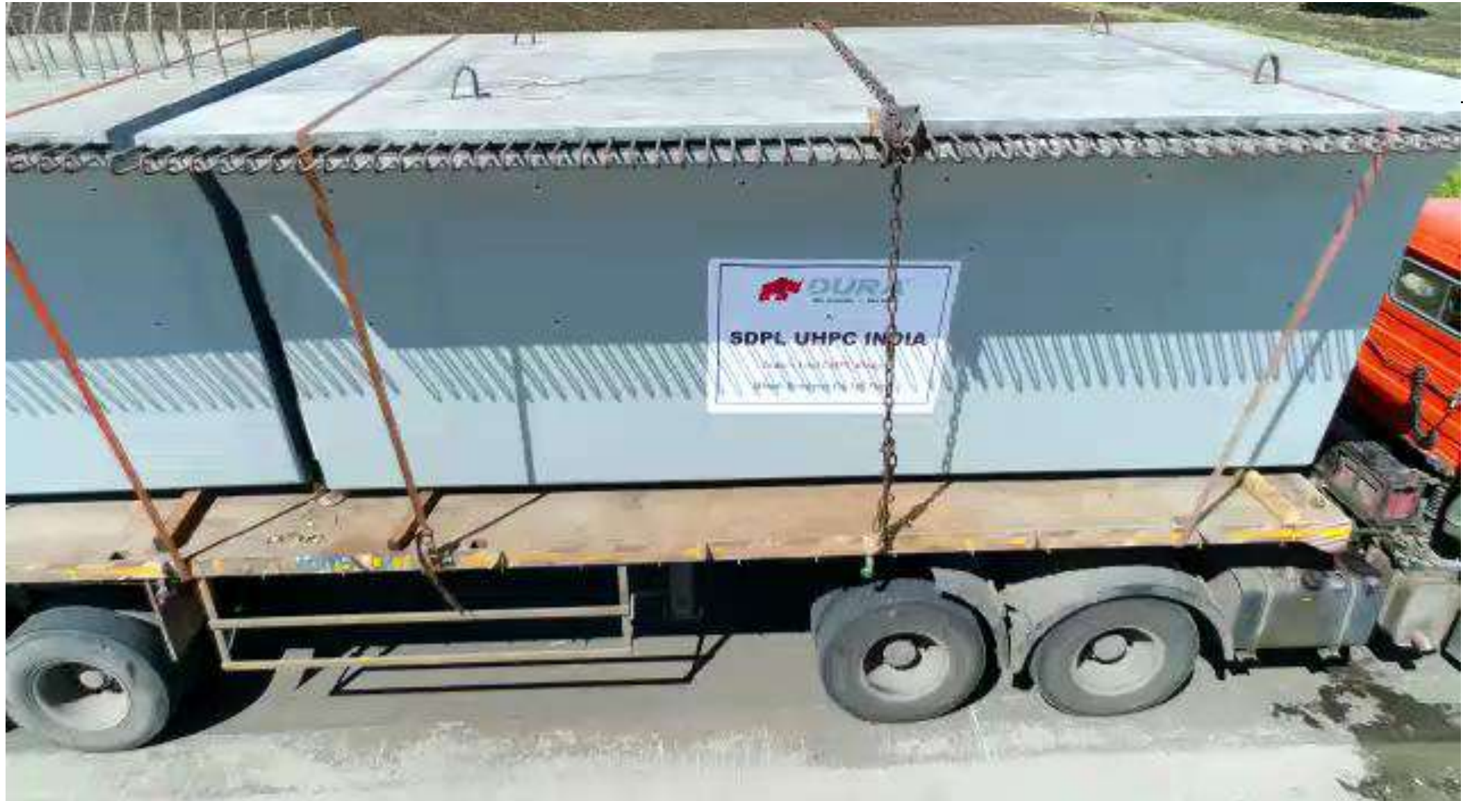
STAGE 1 (b) : ARRIVAL OF SEGMENT ON SITE
